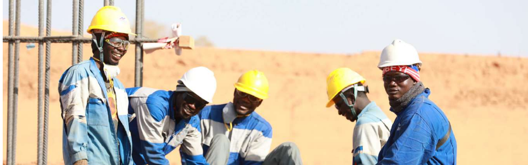
Construction workers on site during expansion activities at the Bomboré Mine.
