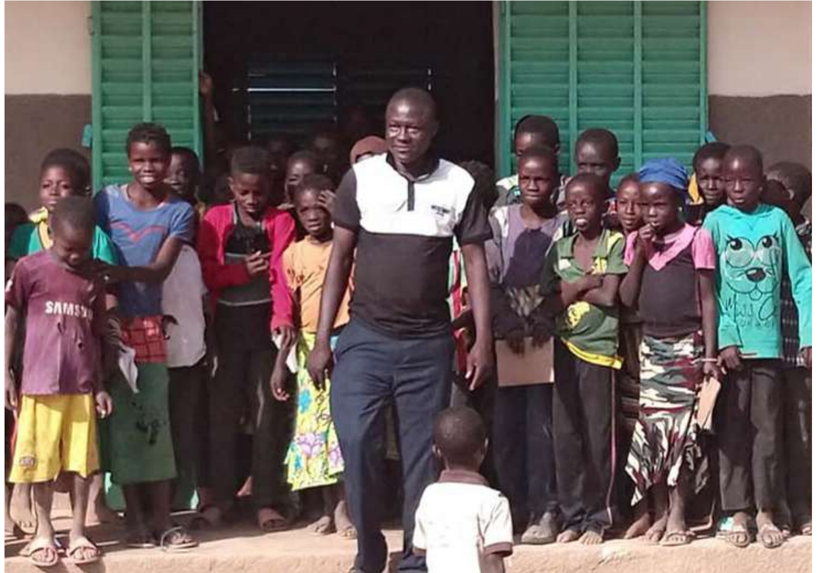
Additional classrooms constructed at the MV2 community, a Government of Burkina Faso and OBSA initiative.
