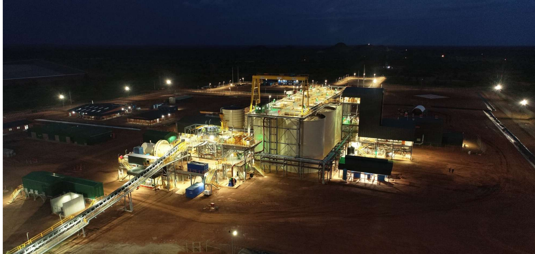
Nighttime aerial view of the Bomboré oxide processing plant.
